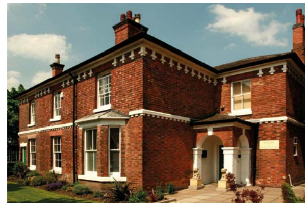
Rehabilitation houses in Burton
